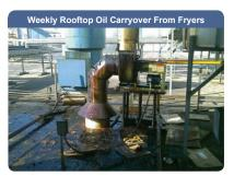
This fryer system was vented straight to the roof, and enough oil collected on the roof to require weekly cleaning, and cause environmental concerns before they contacted Fluid Flow Products about installing a scrubber
